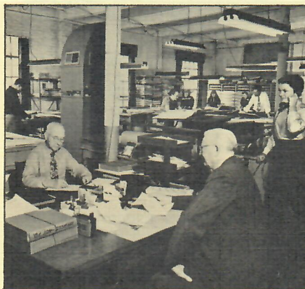
1949 offices CA&E railroad substation
